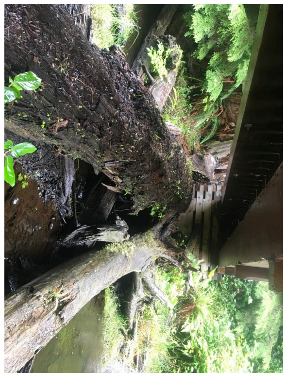
Left Bank Abutment when facing downstream
